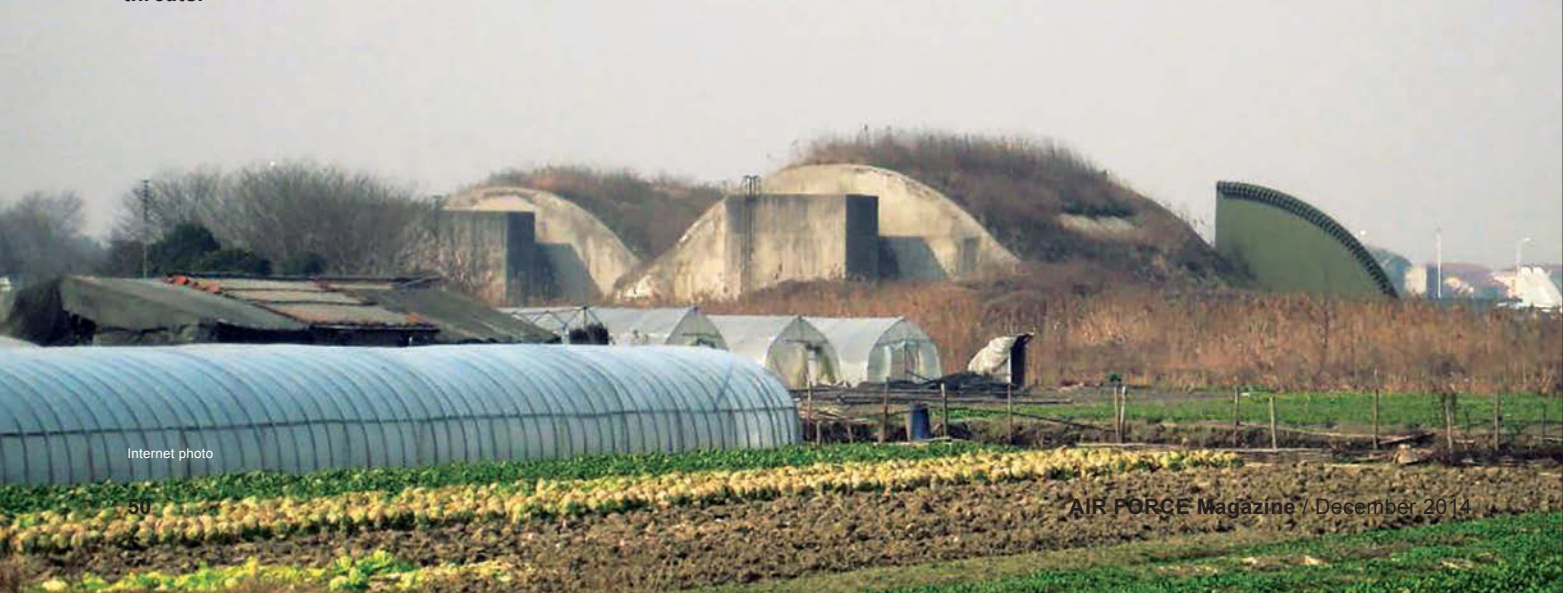
Hardened shelters for China’s Su-30 MK2 fighters. A direct hit by a penetrating bomb could destroy such hangars, but the structures protect the aircraft inside from most other threats.
